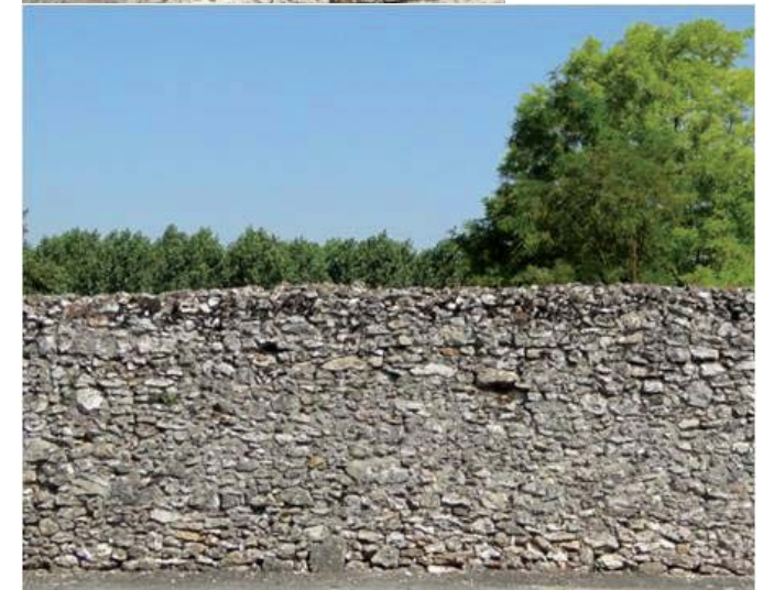
Moellons apparents (calcaire lacustre)
